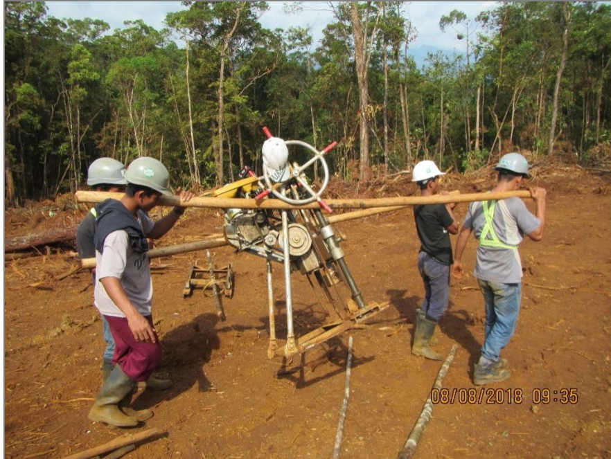
Figure 10-4. Mobilization of drill unit to drill site.
