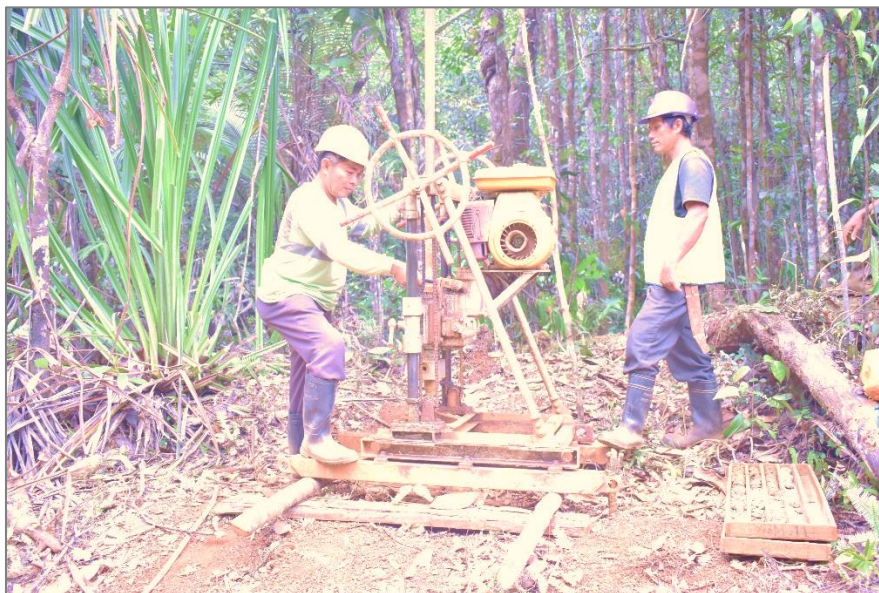
Figure 10-5. MMDC in-house drilling.
