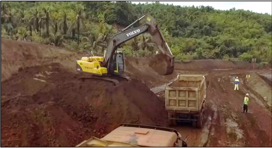
Figure 6-2. Loading of removed topsoil.
