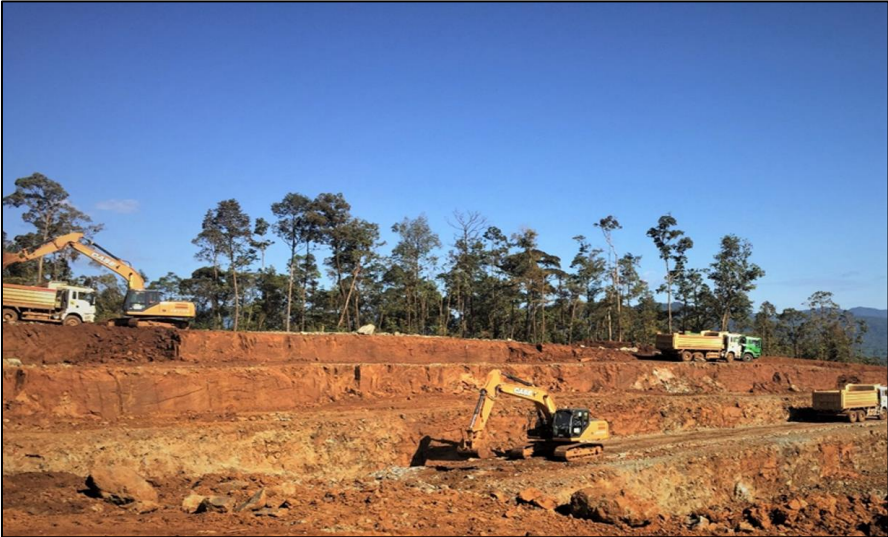
Figure 6-3. Loading of ore to 18-ton capacity dump trucks.
